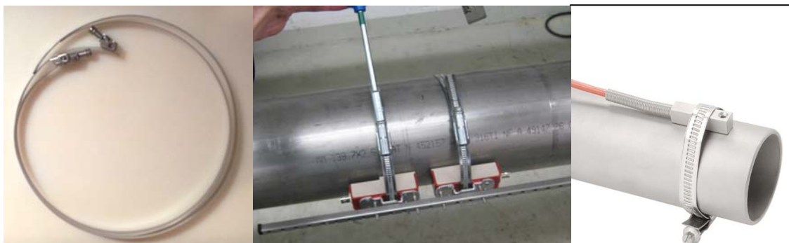
Pictures 10 Mounting US- Transducers, PT100 with stainless steel belts on a pipe
