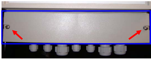
Picture 8 Removing cover plate from cable terminal
